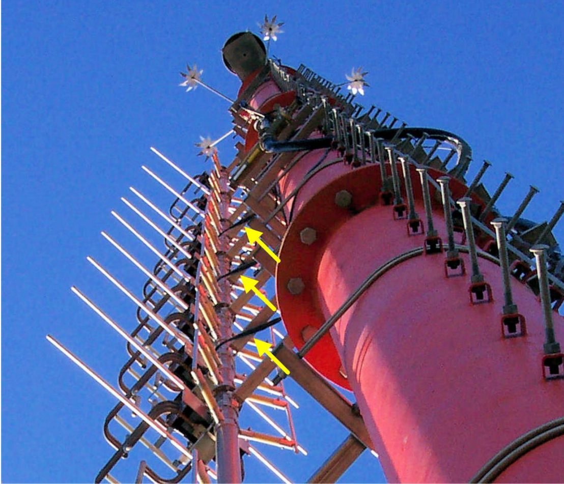
Figure 3. Example of an interleaved antenna which is used to “space combine” the analog and digital portions of an FM IBOC signal. Note that every other bay is fed the analog signal directly by the high power transmission hard-line running vertically behind the bays. The alternate bays are fed the digital signal component by the black coaxial cables running horizontally from the tower to the array (denoted by yellow arrows). Close inspection of the antenna elements reveals that the alternating bays are circularly polarized in opposite directions. (Courtesy of Shively Labs)
