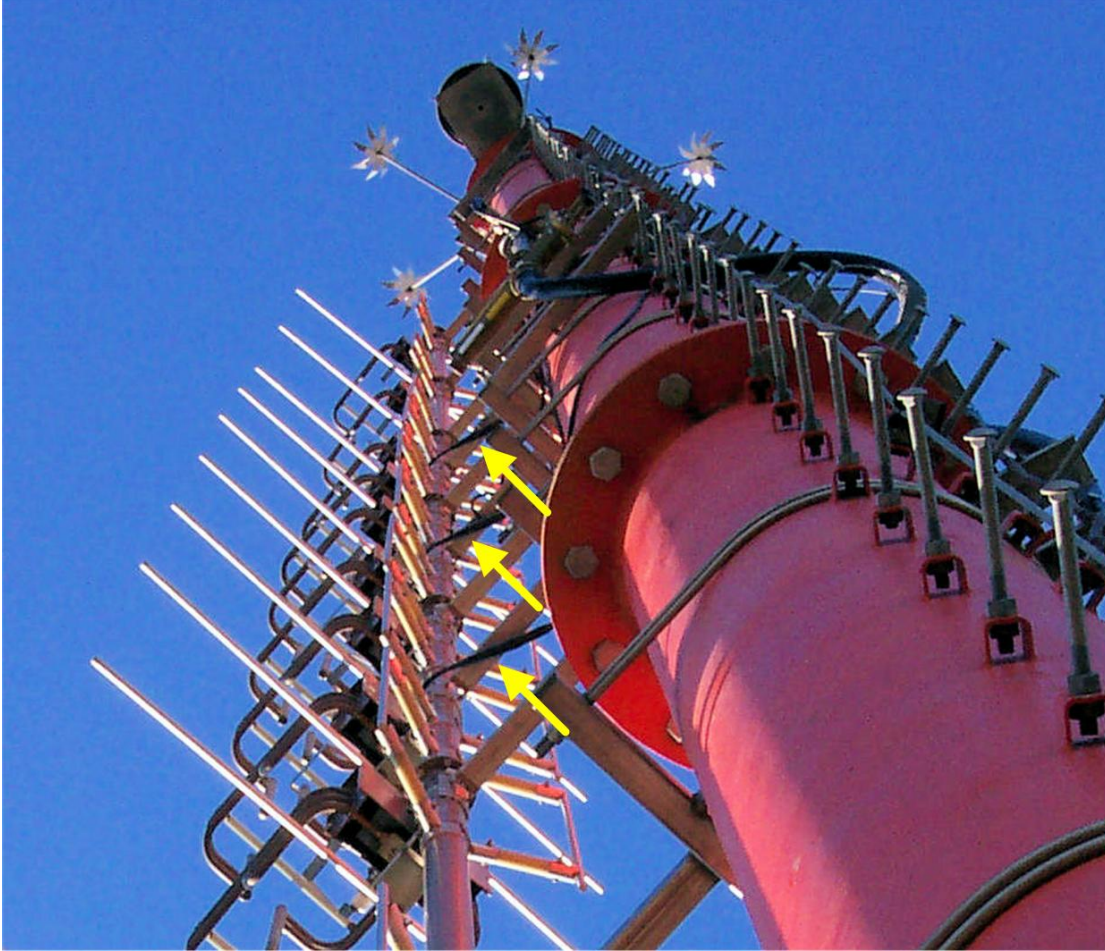
Figure 3. Example of an interleaved antenna which is used to “space combine” the analog and digital portions of an FM IBOC signal. Note that every other bay is fed the analog signal directly by the high power transmission hard-line running vertically behind the bays. The alternate bays are fed the digital signal component by the black coaxial cables running horizontally from the tower to the array (denoted by yellow arrows). Close inspection of the antenna elements reveals that the alternating bays are circularly polarized in opposite directions. (Courtesy of Shively Labs)
